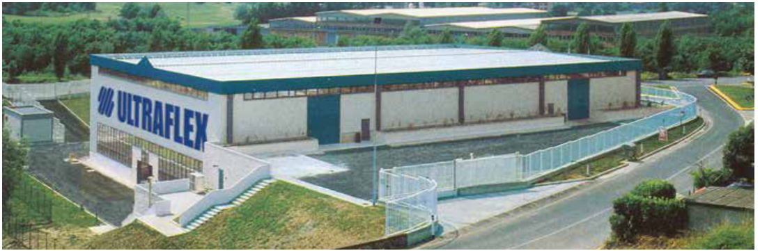
ULTRAFLEX - Factory in Casella
