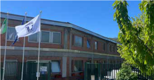
UFLEX & ULTRAFLEX - Headquarter in Busalla
