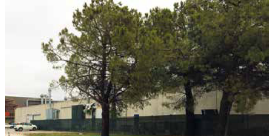
UFLEX - Factory in Tregnago
